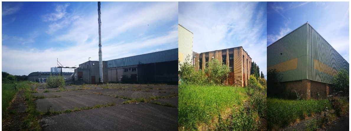
Figure 2.3 – View of the exterior of the existing buildings within the site
