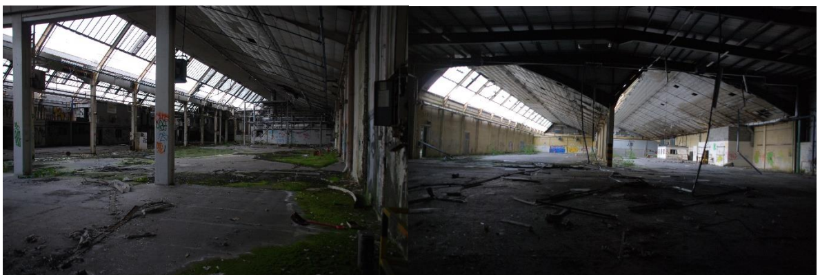
Figure 2.4 – View of the interior of the existing buildings within the site
